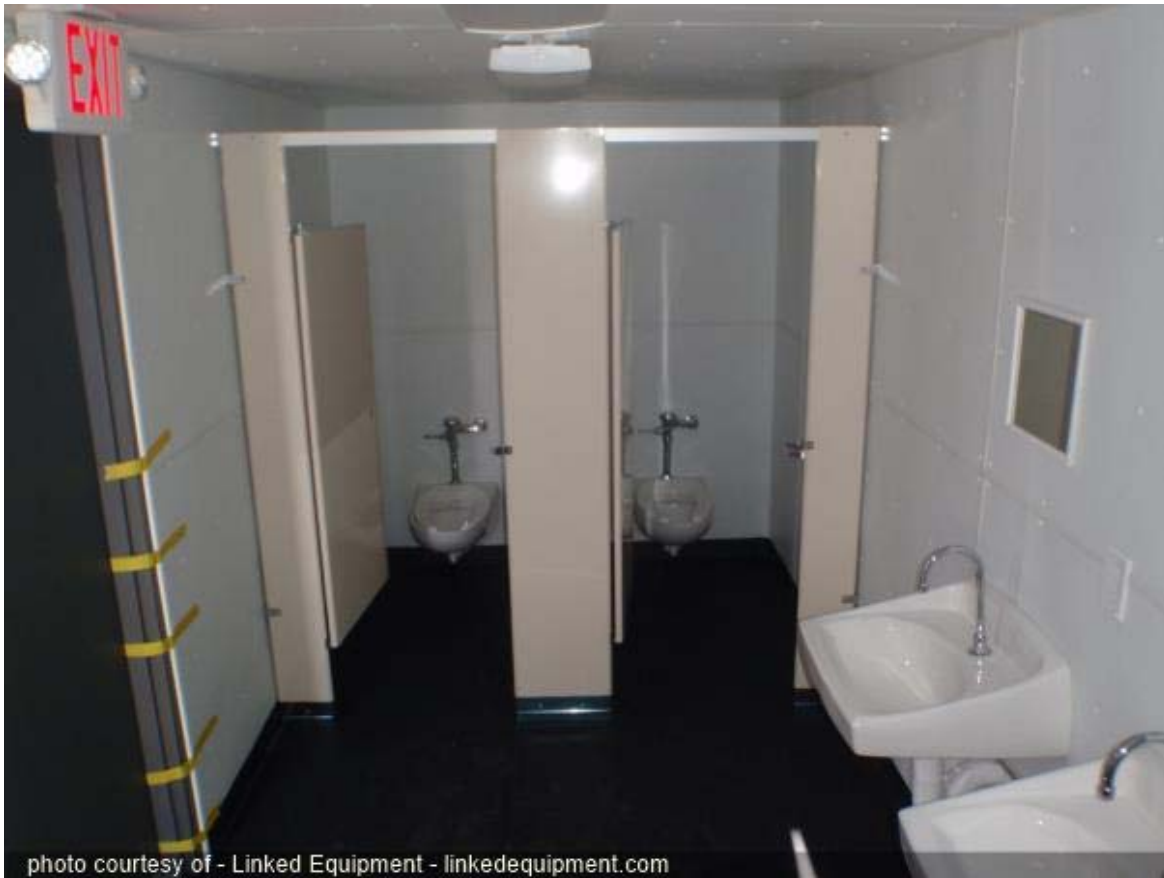
Interior views of Restroom/Shower Facilities.
